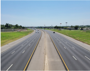
I-35 In Norman From Main St. to Lindsey St.
